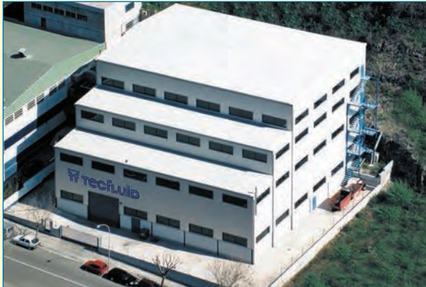
R+D, Manufacturing and assembly workshop
